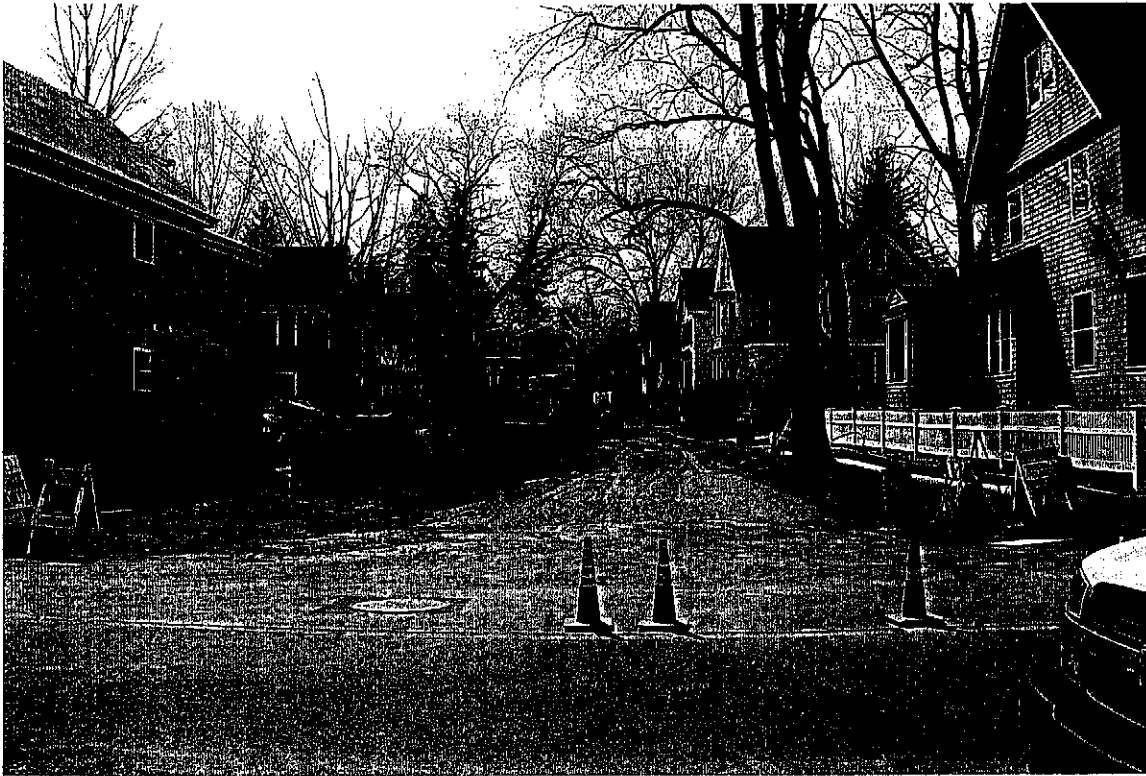
Spring street work area, Facing West.
