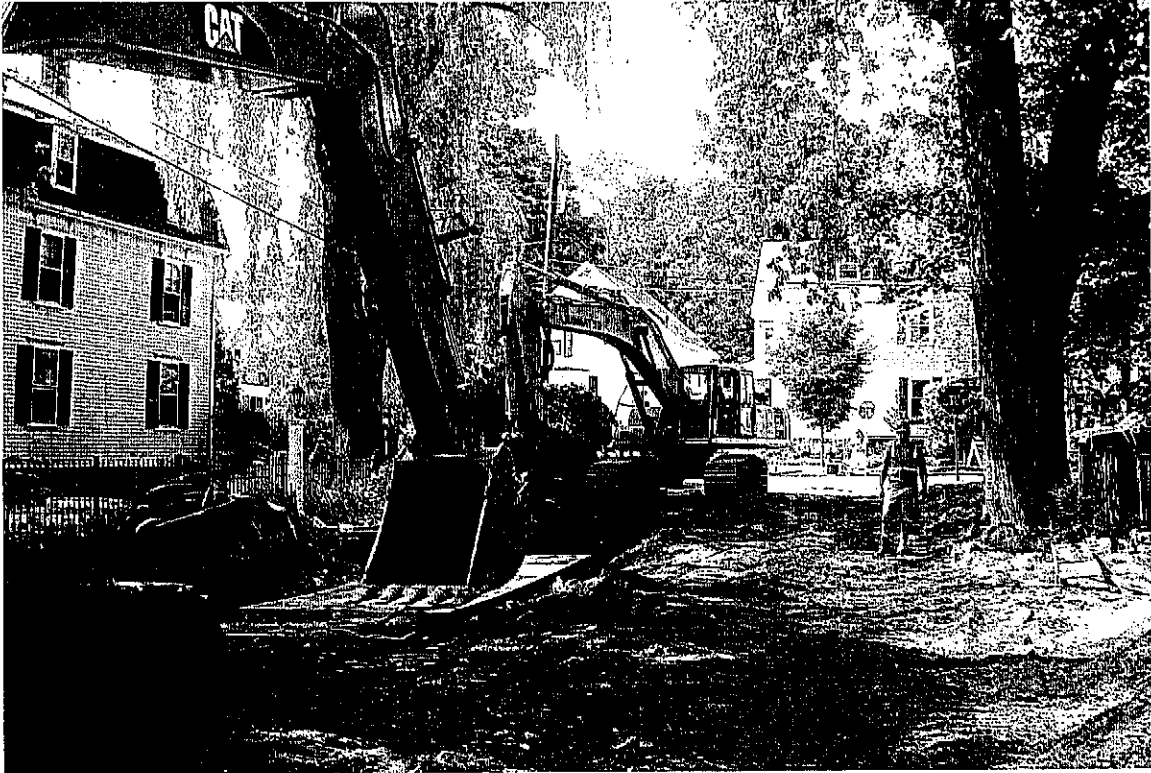
Willow Ln work area facing North
